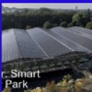
DC car charging park at SS7 NETHERLANDS 2024
